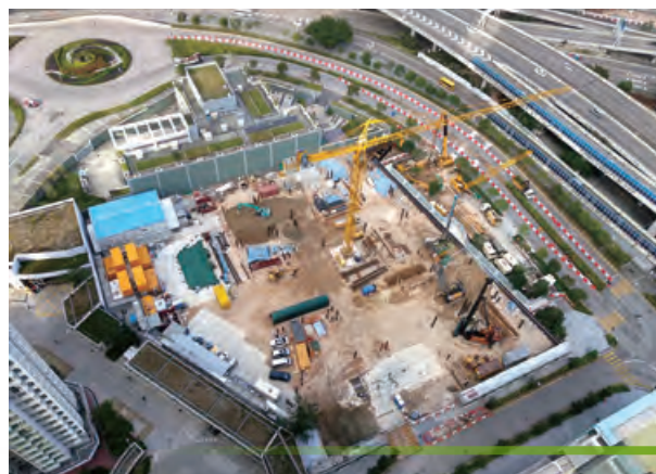
30-classroom secondary school at Site 1A-2, Kai Tak Development 啟德發展區1A-2地盤之一所30班房中學
