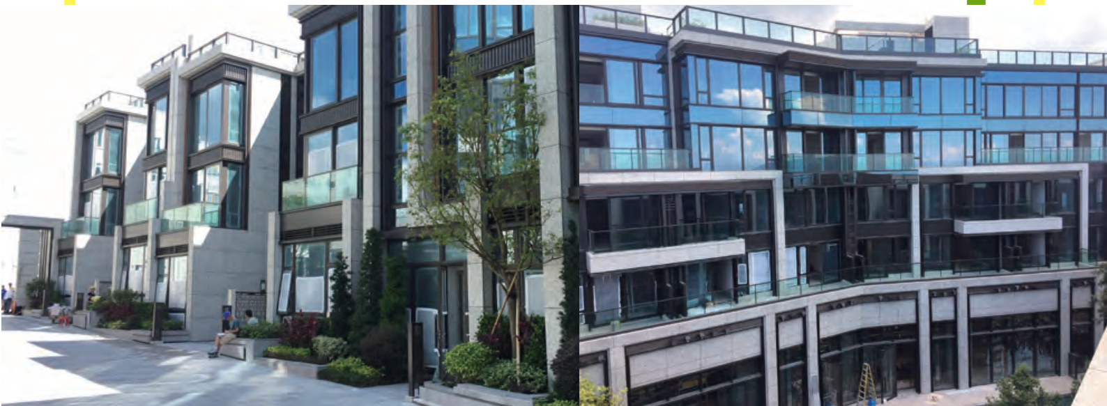
Aluminium window, curtain wall, louver, metal cladding and glass balustrade for St. Moritz at 88 Lai Ping Road, Kau To Shan 九肚山麗坪路88號雲端之鋁窗、幕牆、百葉、金屬飾板及玻璃欄河
