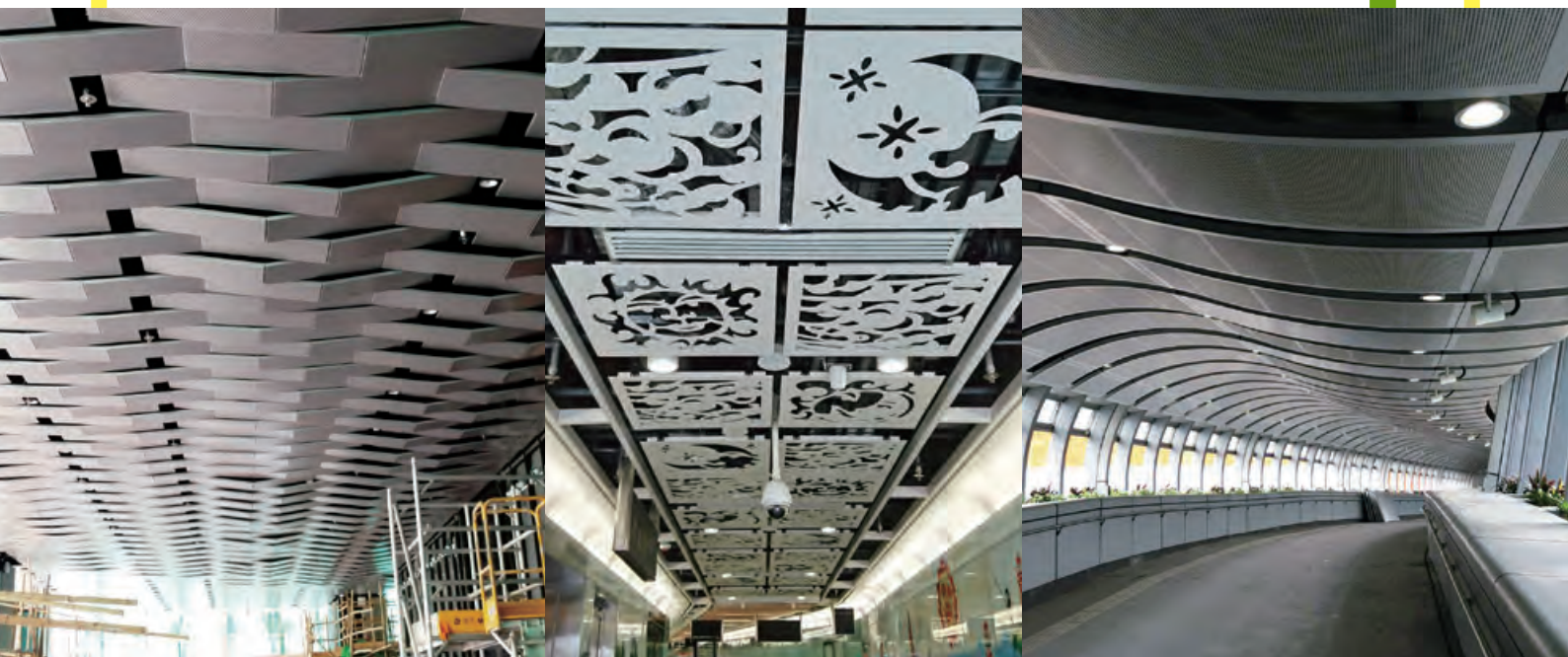
Suspended ceiling system for commercial development at NKIL 6311, MTR's Lei Tung Station and West Kowloon Terminus Station North – Footbridge (from left to right) 新九龍內地段第6311號之商業發展項目、港鐵利東站及西九龍總站(北)項目—行人天橋之假天花系統(從左到右)
